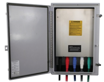
Photo - 2 Distribution Panel and Cam Lock Connections
